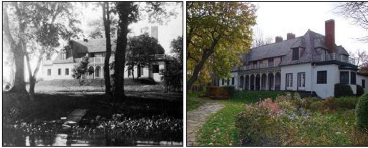
Front (north) elevation of The Stephen Leacock House. Stephen photograph, 1928, Leacock Museum Archives (Public Domain)
